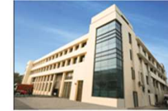
Heat Exchanger Plant
