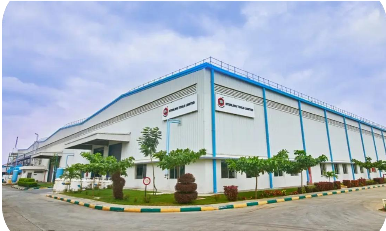
STL fasteners Plant- Bengaluru
