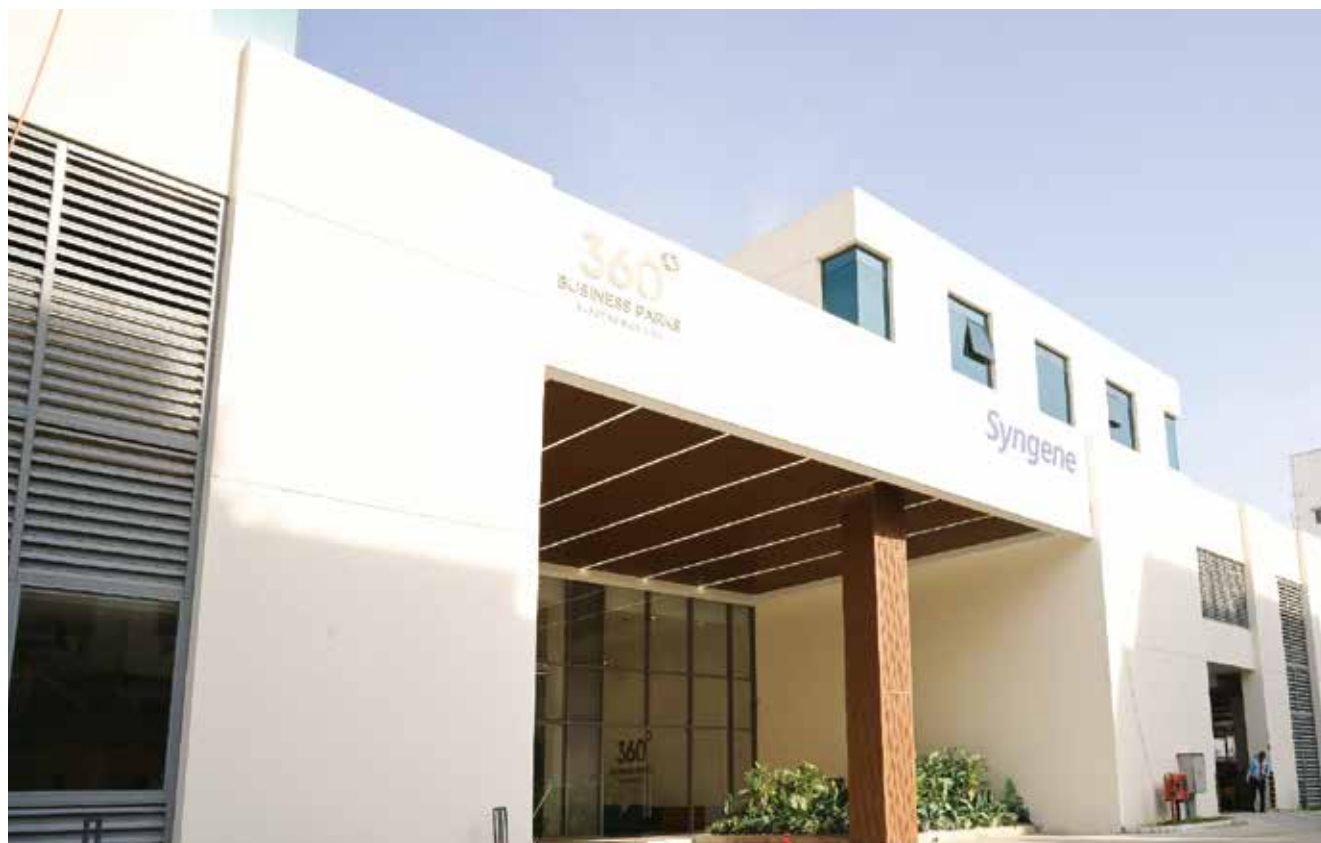
The Hub, housing enabling functions, Bengaluru, India
