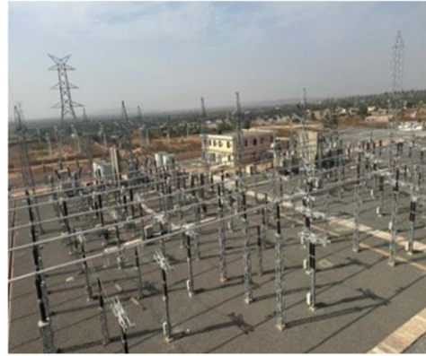
225/30 kV Substation project at Mali
