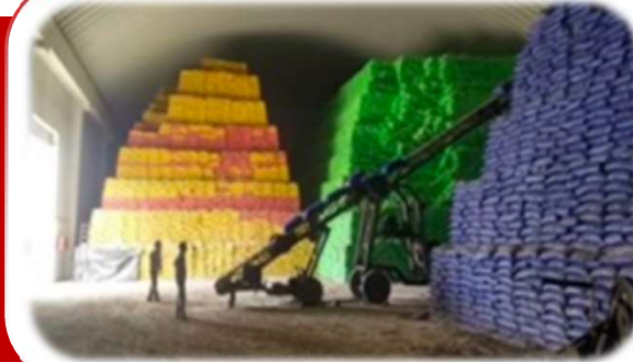
Self-supported roofing structure for a major Indian sugar company at Rajpura, Uttar Pradesh
