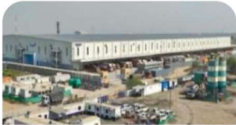
Over 57,000 sq. m. PEB installation for a warehouse, for a multinational e-commerce company at Ahmedabad, Gujarat
