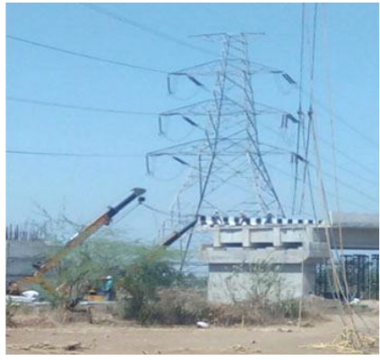
Modification And Upgradation Of System
