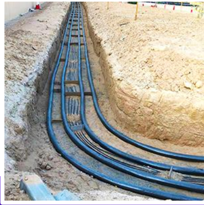
Underground Cable Laying
