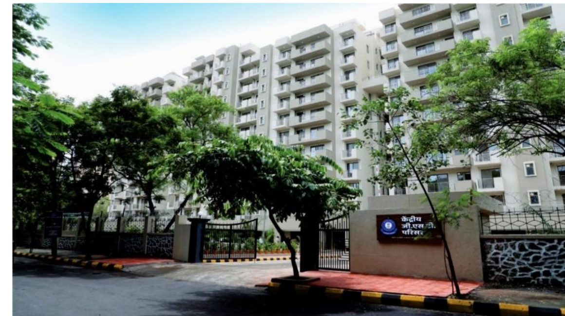
Kendriya GST Parisar, Residential complex at Kharghar, Navi Mumbai Project Cost : Rs. 105 Cr.
