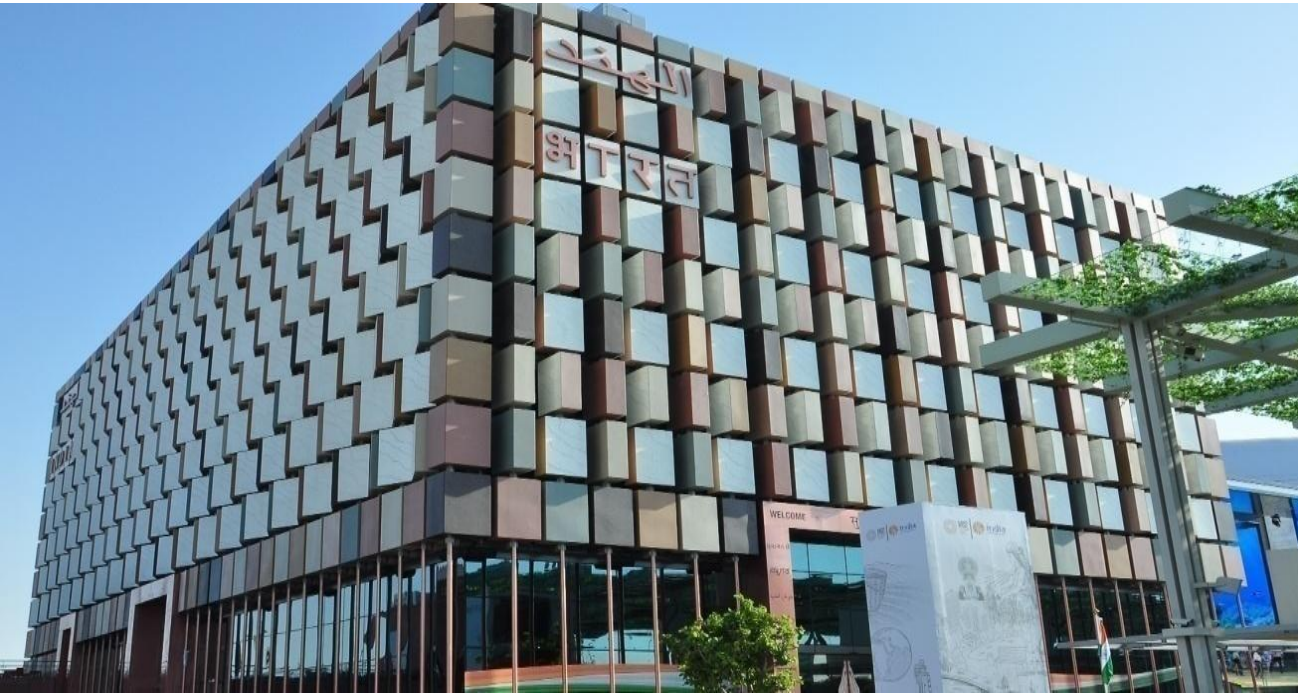
CONSTRUCTION OF INDIAN PAVILION AT WORLD EXPO 2020, DUBAI- USD 46.8 Million/INR 280 Cr.
