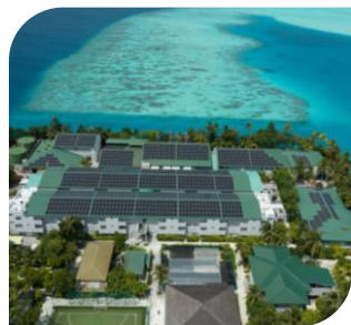
Solar installation, Maldives
