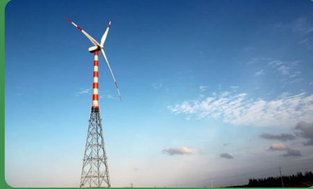
Windmill Lattice Tower
