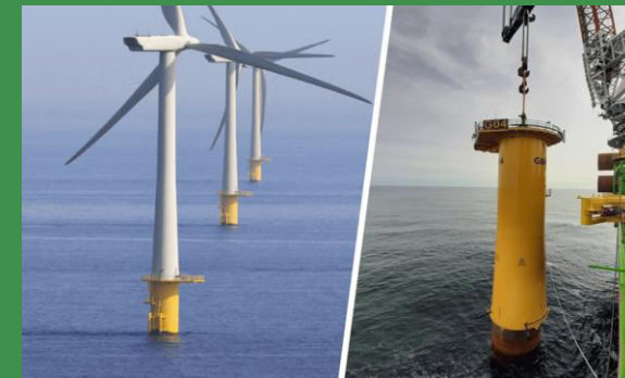
Offshore Tubular Tower
