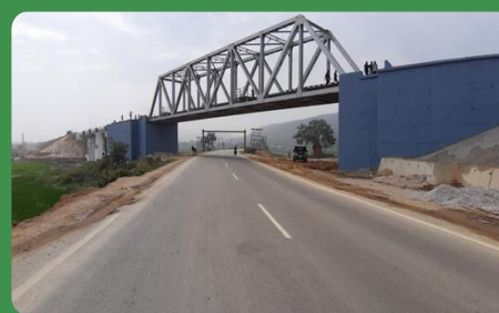
Railway and Highway Bridge
