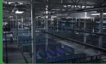
Data Centre Building
