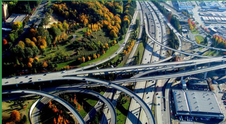
05 Urban and Rural Infrastructure
