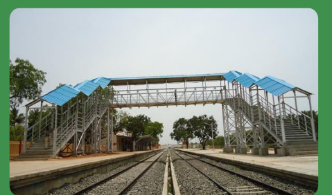
Rail Over Bridge (ROB)
