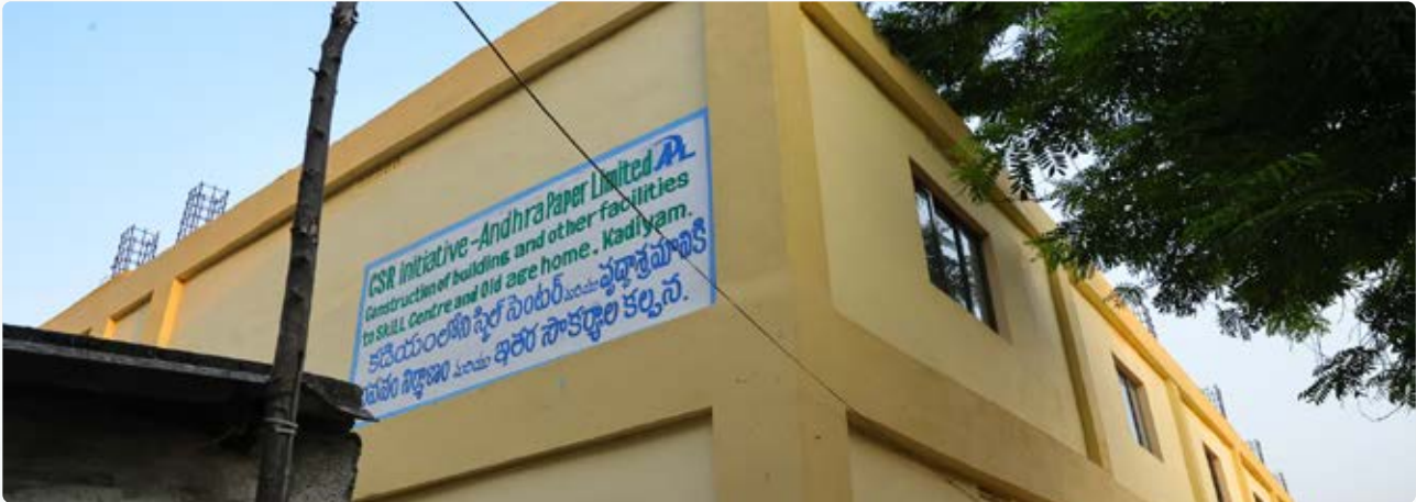
Constructed old-age home and skill development centre facilities at Kadiyam
