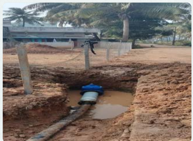
Replaced the 20-year-old pipeline with 550 metres of HDPE pipes at various underprivileged places in Kadiyam
