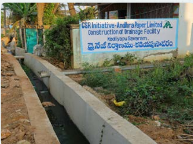
Construction of 500 meters of drainage adjacent to houses to prevent waste water accumulation at underprivileged communities in Kadiyapusavaram
