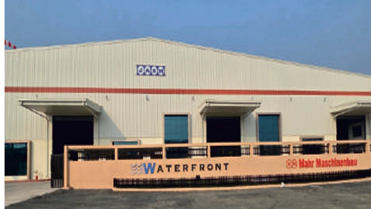
Extension of Stainless Steel Fabricated Product Plant - SEZ, Pithampur
