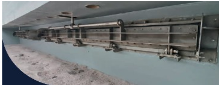
Super Duplex Tilting Flap Gate / Valve for Desalination Plants
