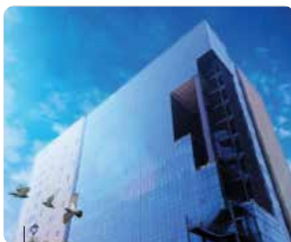
Data Centre, Panchkula
