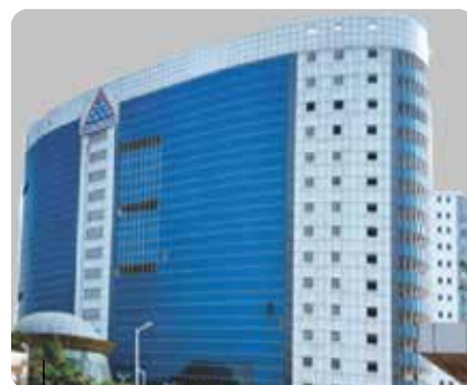
Data Centre, Rai
