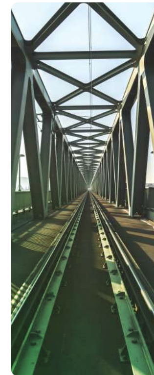
Railway Over Bridge (ROB)
