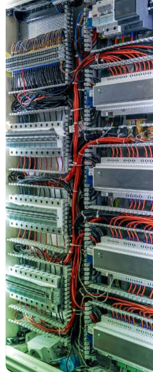
Cable Tray & Earthing Material
