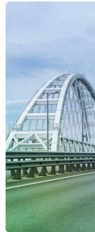
Railway and Highway Bridge
