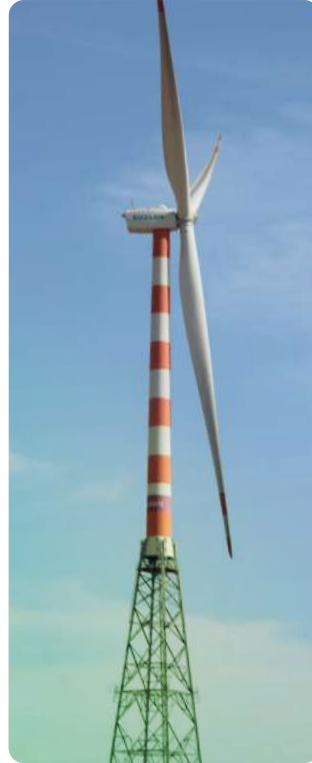
Windmill Lattice Tower
