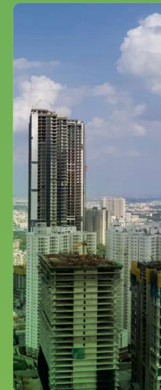
Urban and Rural Infrastructure
