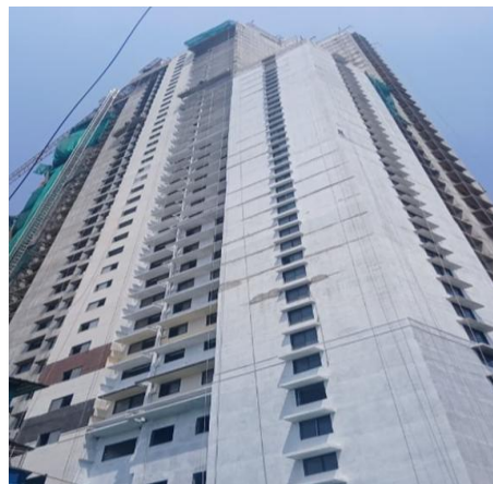
MUMBAI METRO HIGH-RISE BUILDING
