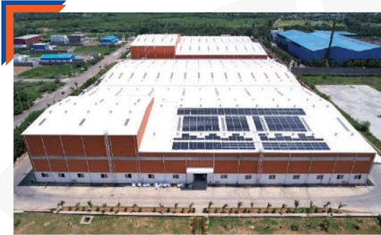
Vizag Plant (Capacity: 150 KWP)
