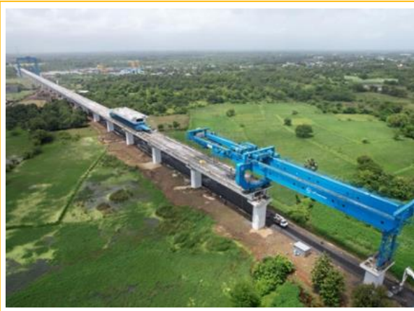
Mumbai Ahmedabad Bullet Train [Chemicals & Aggregate Supply]
