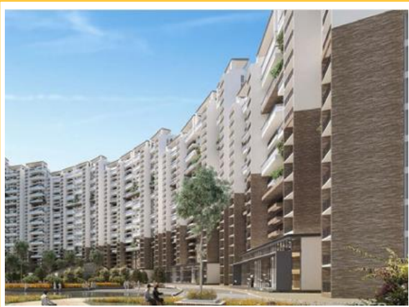
Listed Developer Project, Whitefield Bangalore [Aggregate Supply]
