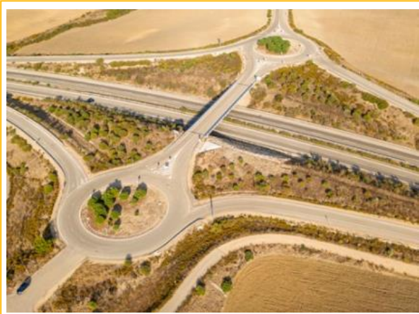
Chennai Peripheral Ring Road [Aggregate supply]
