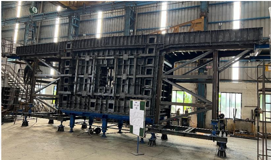
Pier Head Segment
