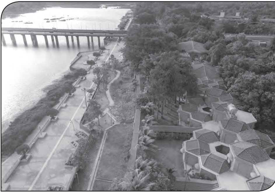
RAS BY TREAT-AERIAL VIEW
