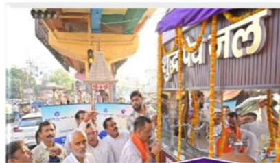
Installation of Water ATM
