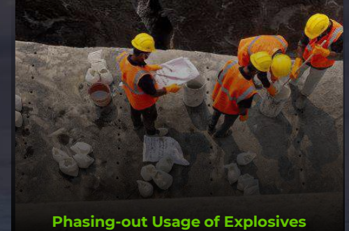
Phasing-out Usage of Explosives
