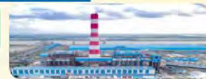
BIFPCL 2x660 MW Thermal Power Plant, Bangladesh
