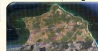
120 MW Solar Project in Sri Lanka
