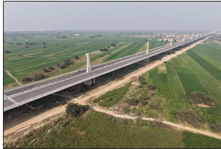
L&T Daewoo- Patna Bridge
