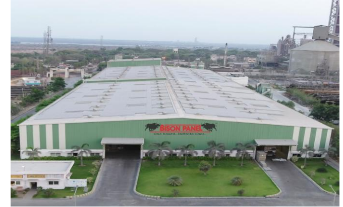
Plant 3 – Simhapuri (Unit III) Location: Suryapet, Telangana Capacity: 30,000 MT
