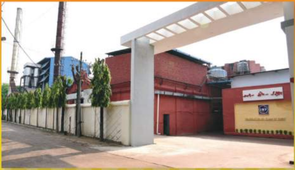
Plant at IZZATNAGAR, Barielly
