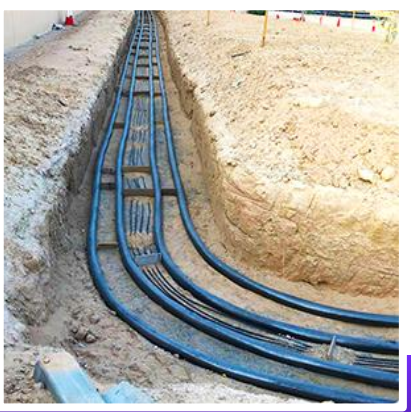
Underground Cable Laying
