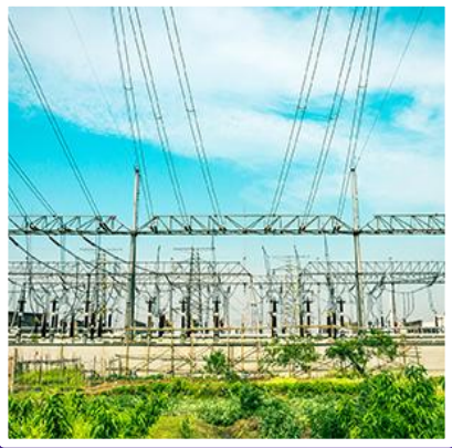
Liasoning With Govt. Authorities And Utilities
