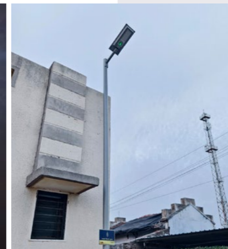
Solar street lights in Manipura, Ahmedabad. 147 lights being installed at 70-metre intervals across the village, reducing grid dependence and improving community safety.
