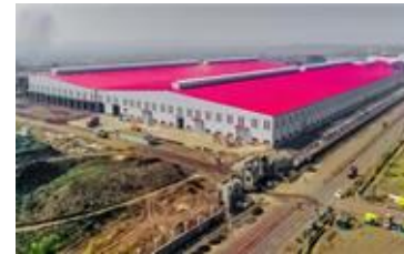
Pre-engineered Steel Buildings
