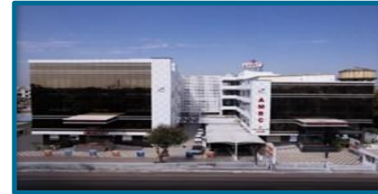
Amar Hospital and Research Centre, Jaipur , Feb 2022 (250 beds)
