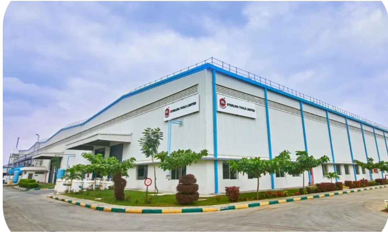
STL fasteners Plant- Bengaluru
