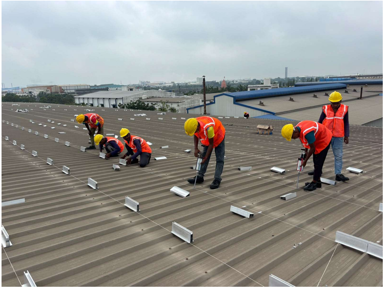
Photograph 1 - On-site execution team carrying out rooftop marking and mounting-structure related work. The image shows active installation activity across the industrial roof.
