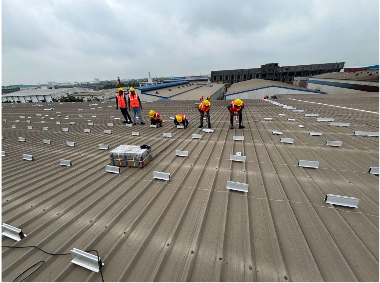
Photograph 2 - Wider rooftop view showing multiple MMS work fronts and installation personnel deployed across the project area.
