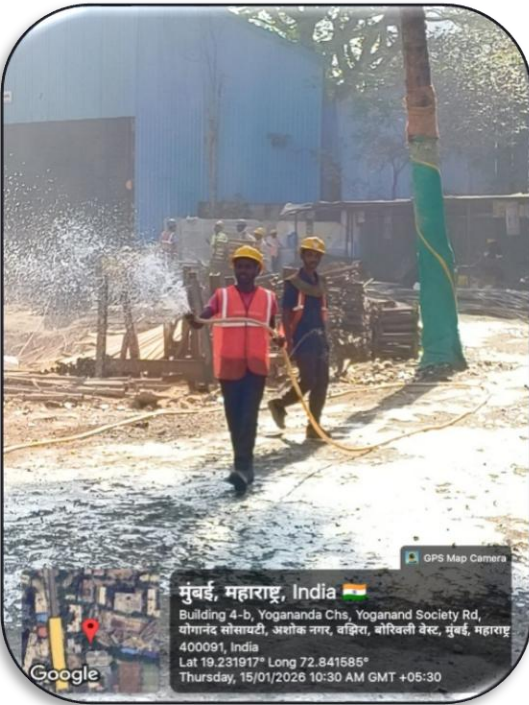
Water spraying for dust suppression
