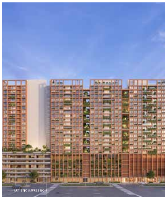
CREST GREENS PHASE III RAIPUR, CHATTISGARH
