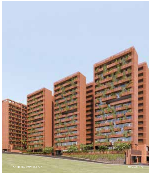
CREST ASPEN ANDHERI, MUMBAI
