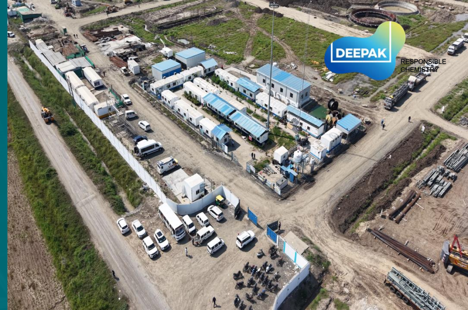
DCTL D3 Site office
