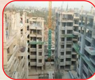
Significant progress on civil structure front
