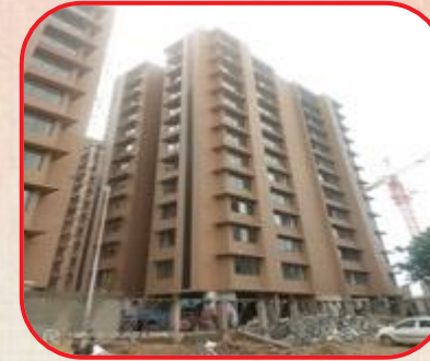
Structure work completed in all towers
