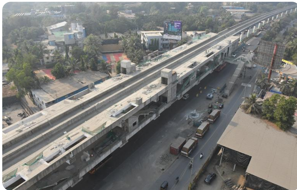
MUMBAI METRO LINE 4A
