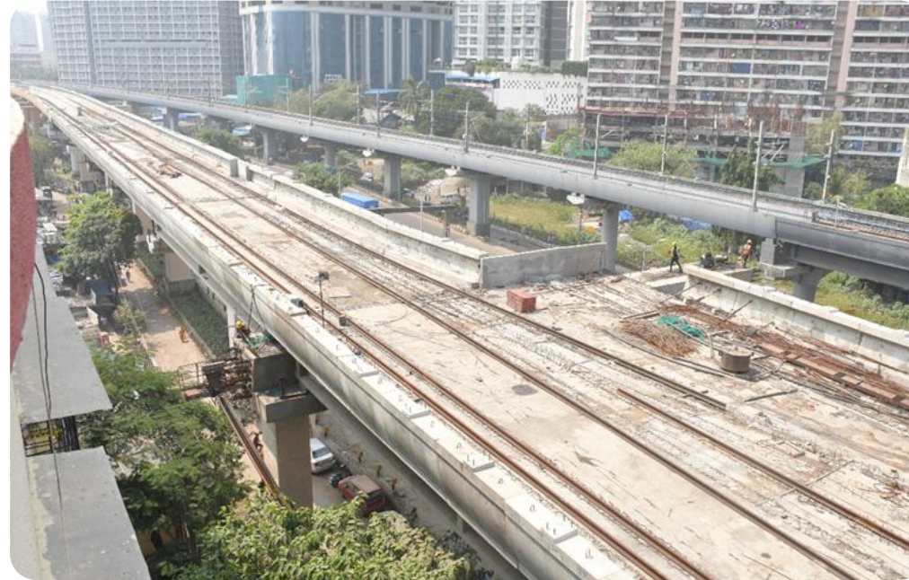
MUMBAI METRO LINE 9
