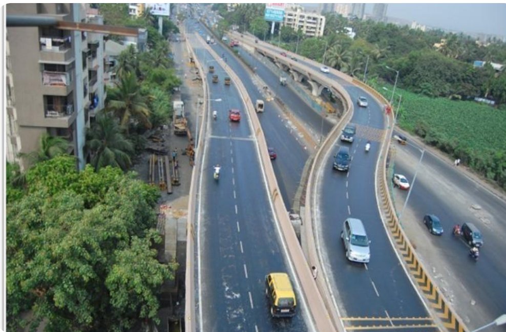
AMAR MAHAL FLYOVER
