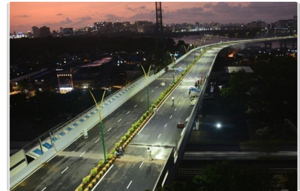
BKC- CHUNABHATTI FLYOVER
