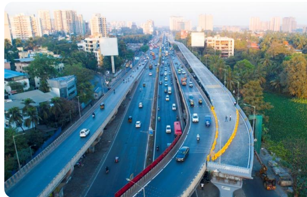
CHHEDA NAGAR FLYOVER PART 1
