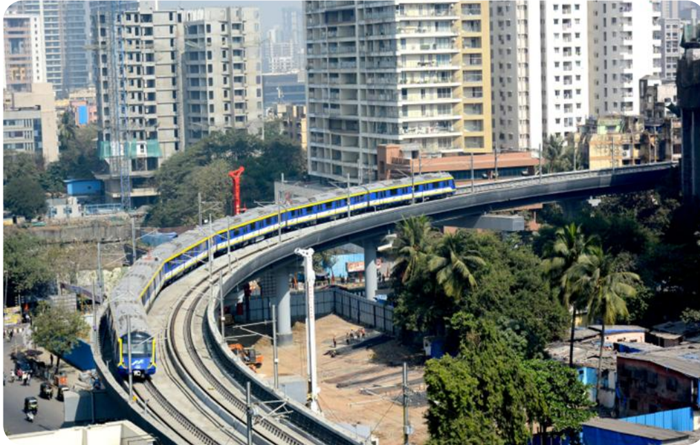
MUMBAI METRO LINE 2A
