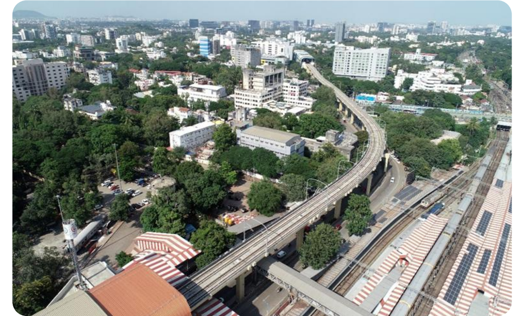
PUNE ELEVATED METRO
