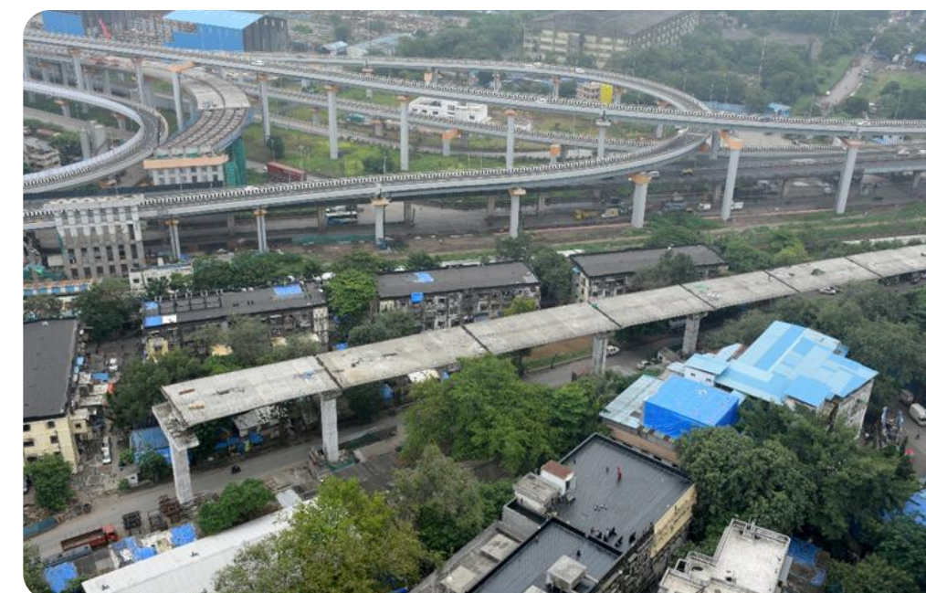
SEWRI WORLI ELEVATED
