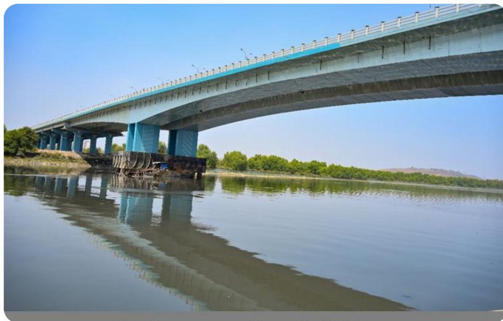
MOTAGAON CREEK BRIDGE
