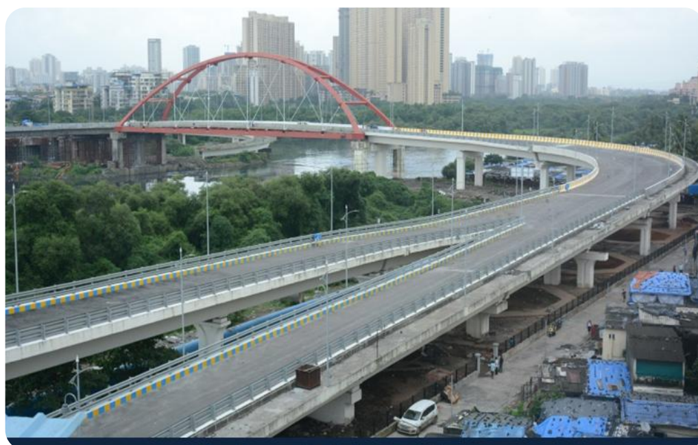
KALWA BRIDGE THANE
