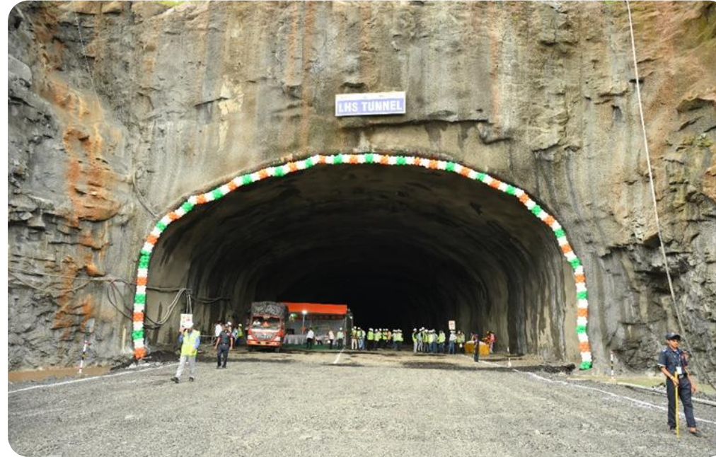
VADODARA MUMBAI EXPRESSWAY, IRCON
