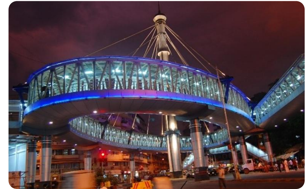
GRANT ROAD SKYWALK
