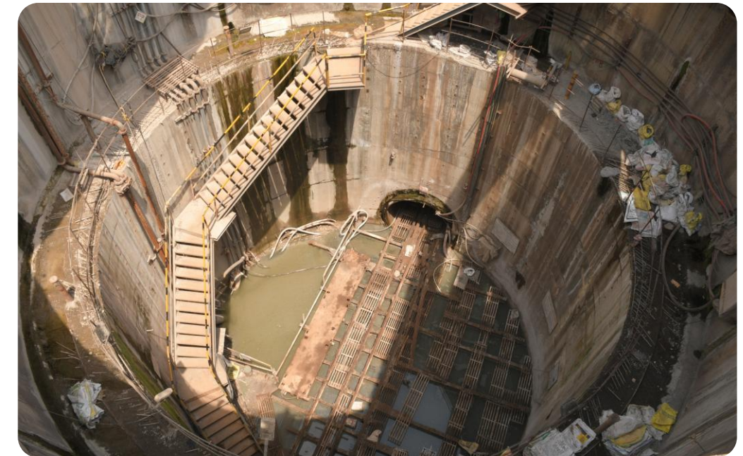
SEWERAGE PROJECT, MALAD
