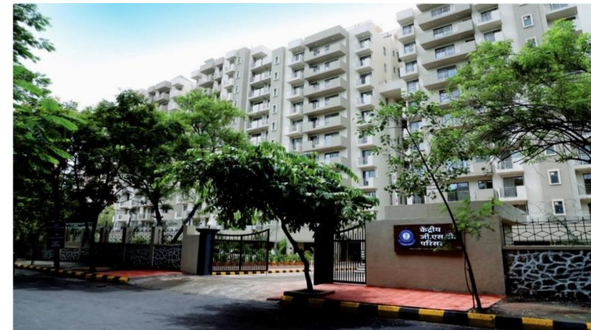
Kendriya GST Parisar, Residential complex at Kharghar, Navi Mumbai Project Cost : Rs. 105 Cr.
