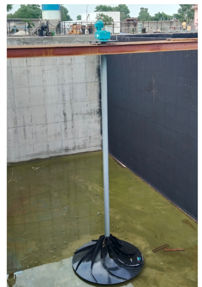
Hyperclassic Mixer Suitable for Tank Size 32.5m (L) X 8.8m (W) X 7m SWD + 0.5m FB
