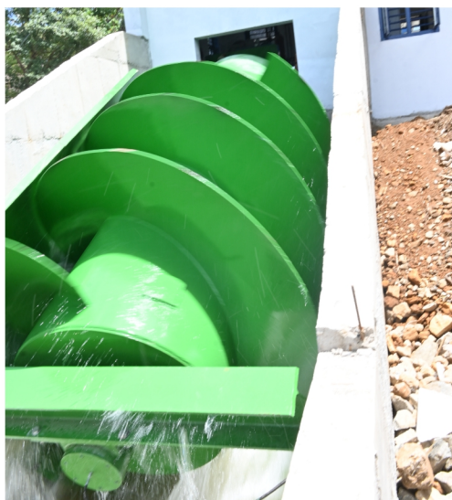
1x36 kW Archimedean Screw Turbine
