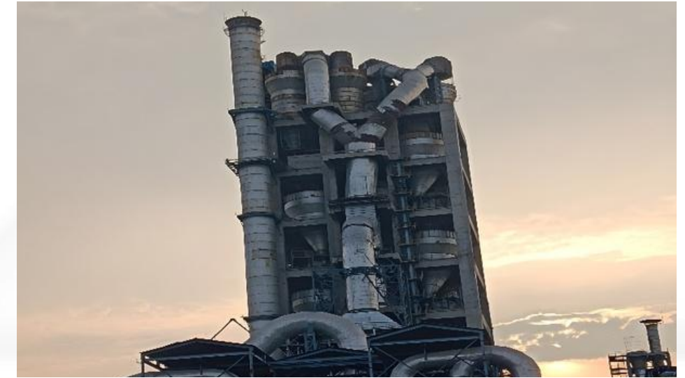
Order Size: 109 Crs Completed Year: 2023 Segment: Cement Plant State: Chattisgarh
