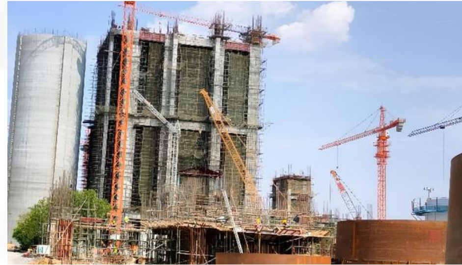
Order Size: 113 Crs Completed Year : 2024 Segment : Cement Plant State: Rajasthan
