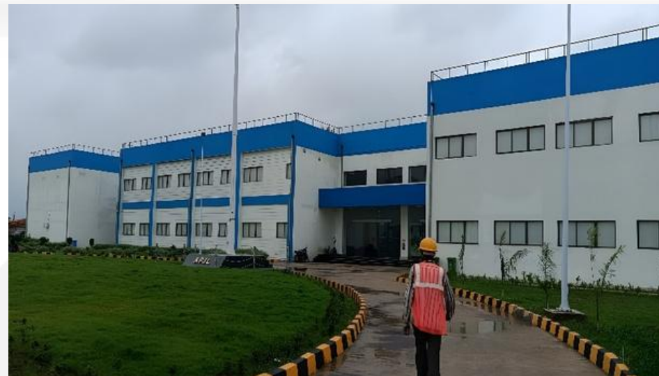
Order Size: 102 Crs Completed Year : 2023 Segment: Power Plant State: Jharkhand
