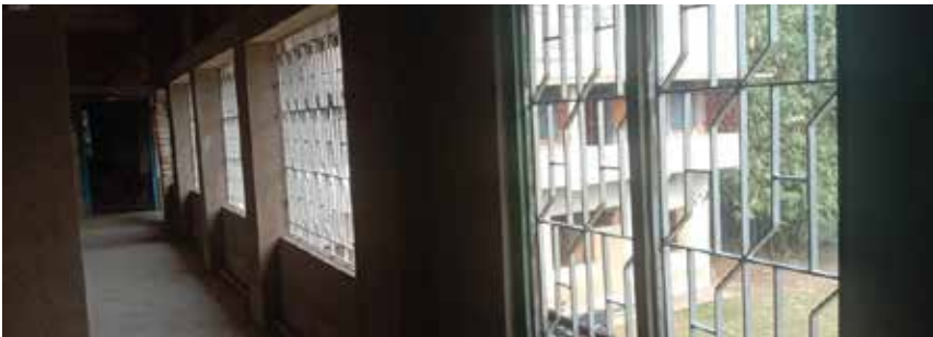
School Building Programme
