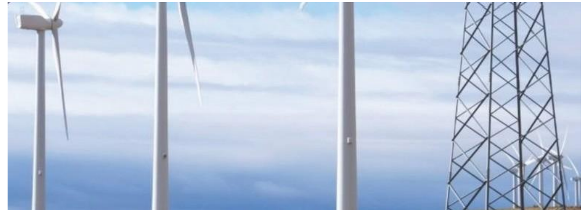
Khavda Renewable Energy Park AL-59 conductors for the world's largest RE hub
