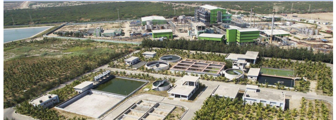
Mundra Petrochem Limited (Adani Enterprises Ltd) Powering India's landmark 1 MMTPA Green PVC plant of Mundra Petrochem.
