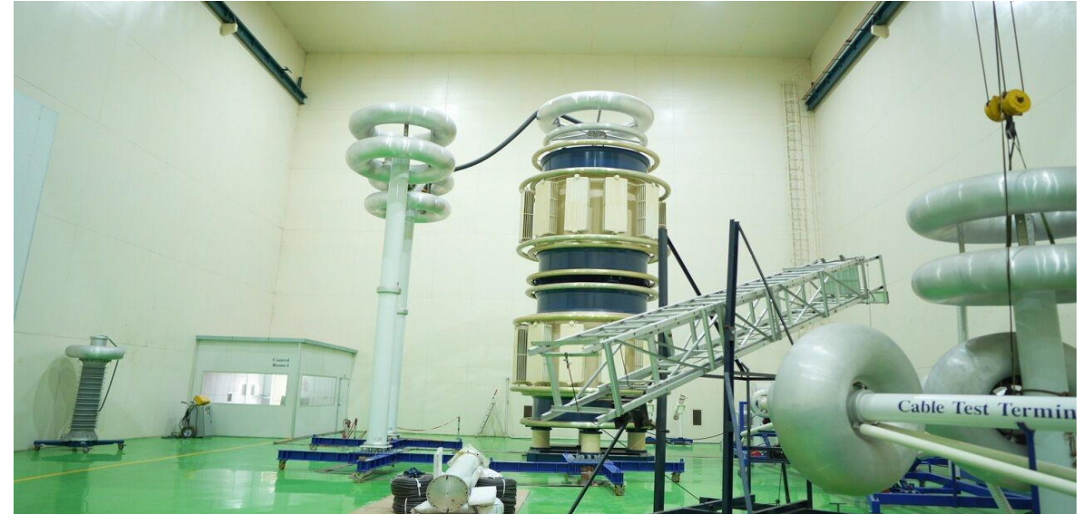
High-voltage & partial-discharge test bays
