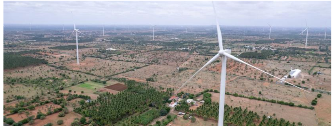
TATA Power Renewable Energy Limited 302.4MW Bijapur -KA Wind project.
