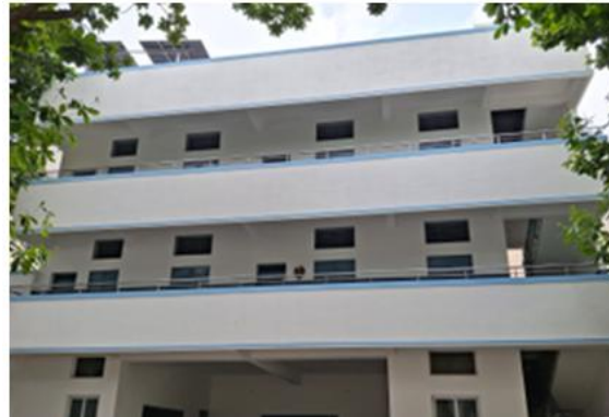
Construction of Government school building
