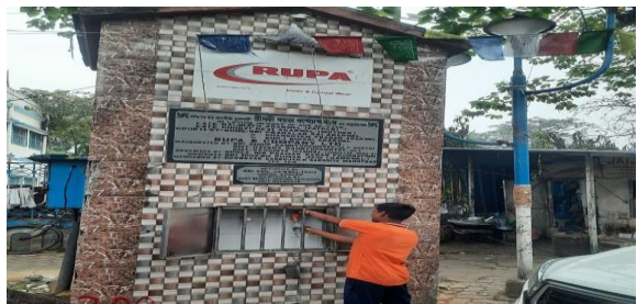
Drinking water facility
