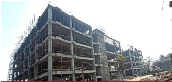
Medical and healthcare facility under construction
