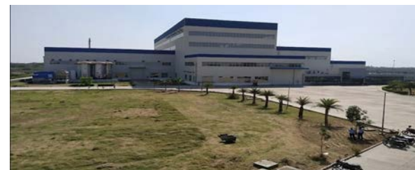
Atlanta Trafo Limited* (100% Subsidiary)
