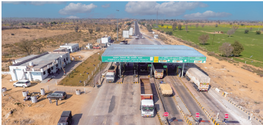
Roads and highways infrastructure - Construction projects
