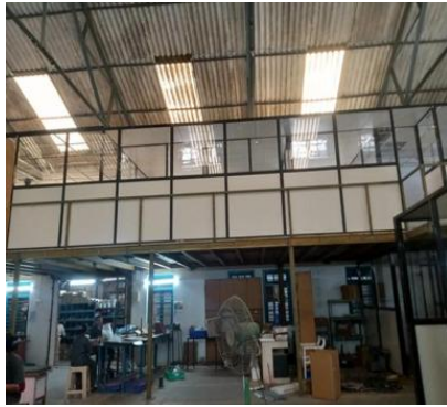
Electrical Component manufacturing unit at Nashik, Maharashtra
