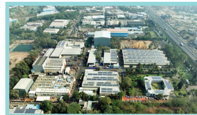
Switchgears Manufacturing Facility Nashik, Maharashtra
