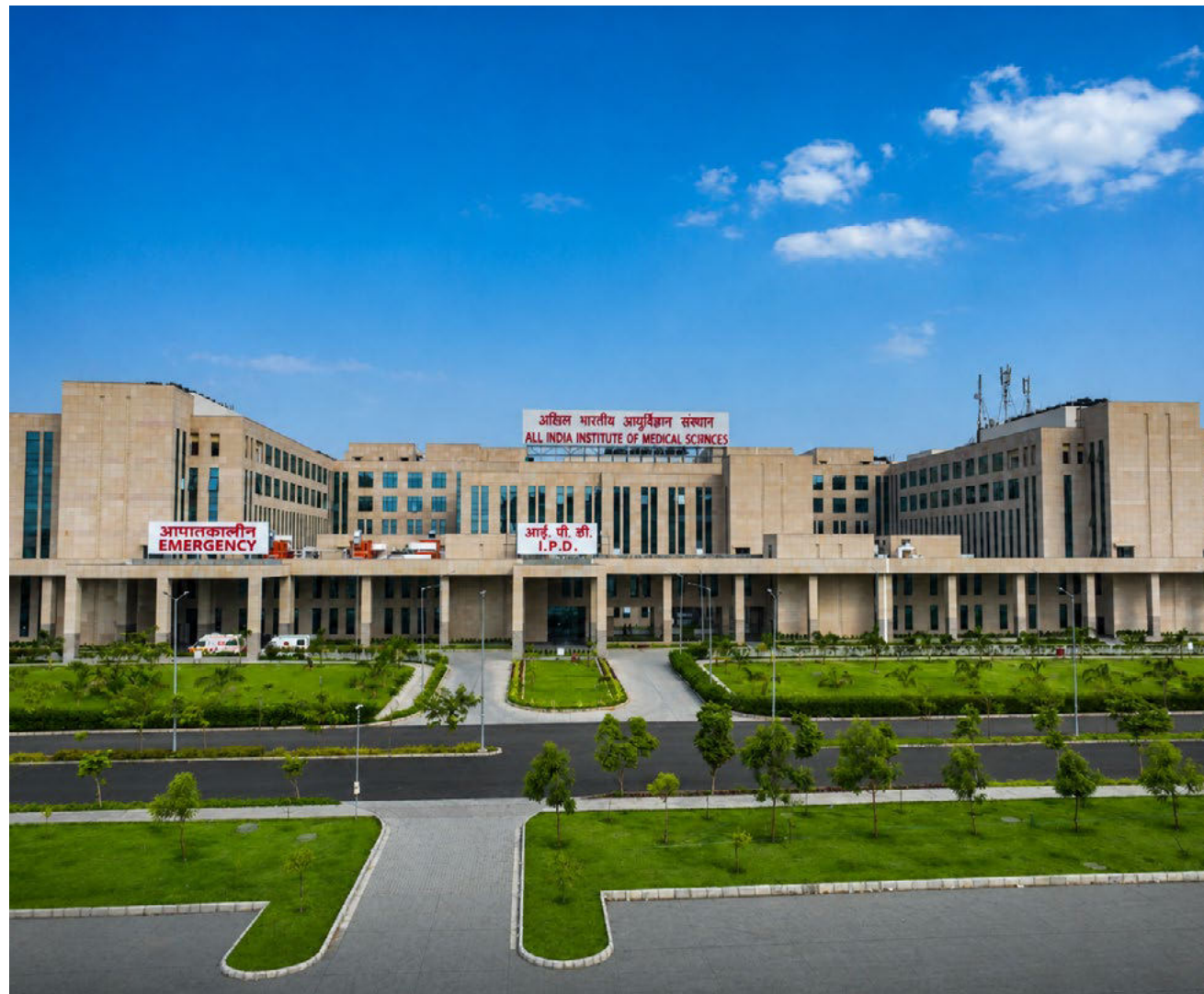
UMPESL Project at AIIMS Nagpur
