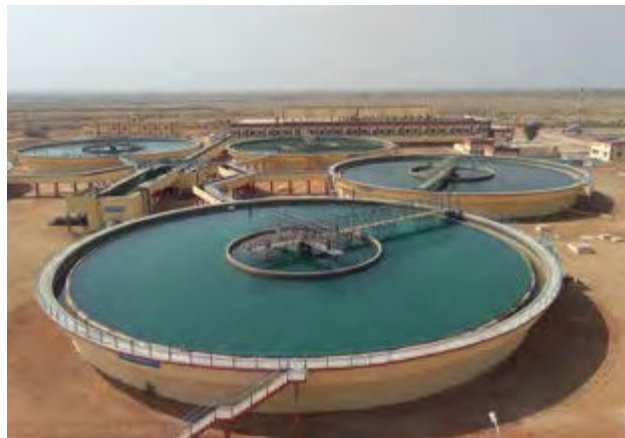
Water Treatment Plant at Uttar Pradesh
