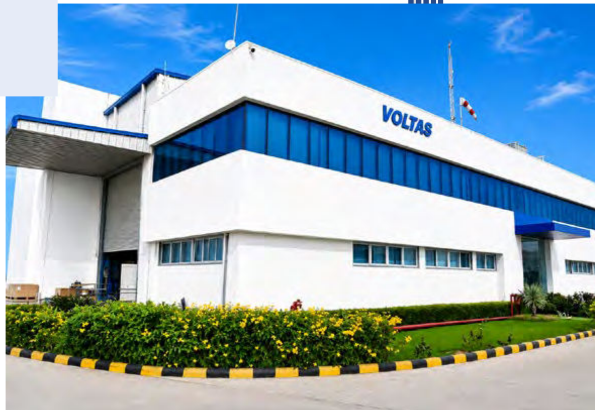
Waghodia Factory Premises
