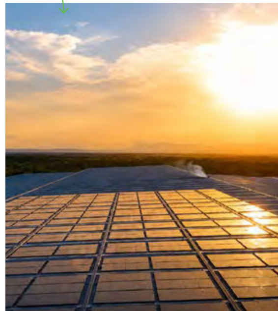
Solar Installation by Voltas
