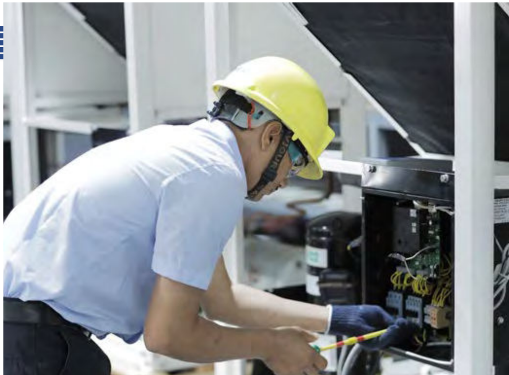
Voltas Technician at Work
