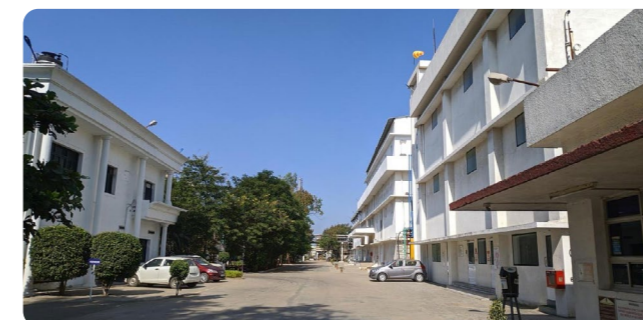
State-of-the-art D9 US FDA accredited API facility at Panoli, Gujarat
