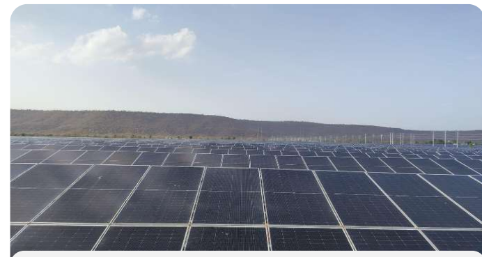
255 MWp Neemuch, Madhya Pradesh 1
