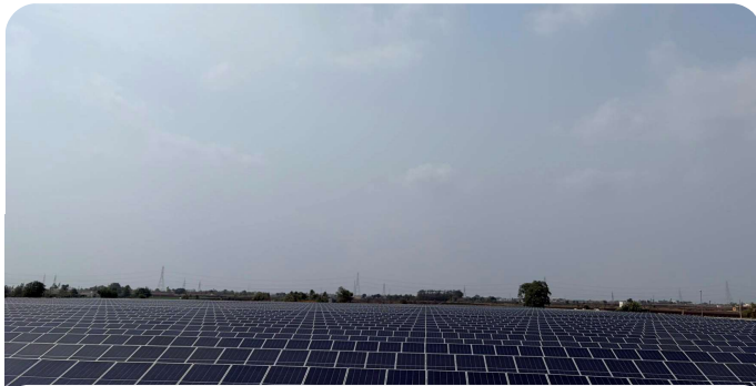
105 MWp Jamnagar, Gujarat 1
