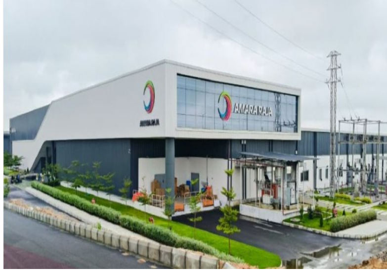
Pack Assembly Plant- Mobility- Divitipally Capacity ~ 1.5 GWh
